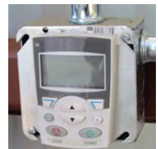
Keypad relocated to 4x4 electrical box
